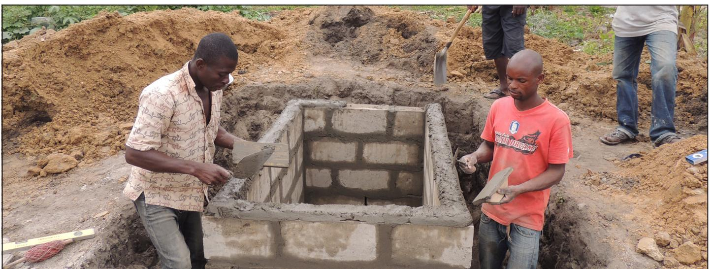
Pits dug in loose soil must be encased with walls to prevent cave-ins and flood damage. Traditionally, these walls are made from concrete cinder-blocks, and the installation process is expensive and requires specialized labor, tools, and time.
