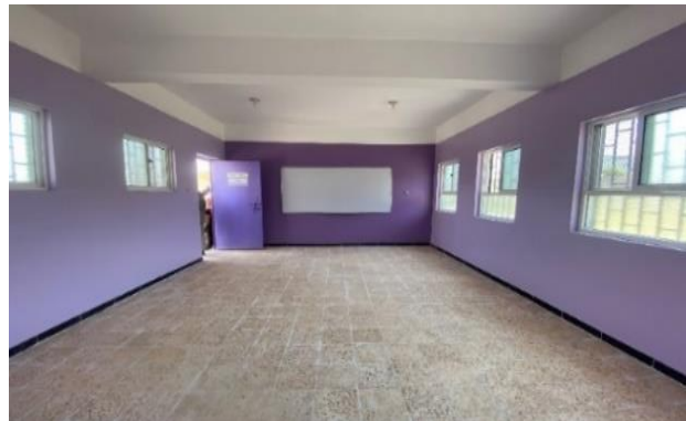
Image: One of the rehabilitated classrooms at the Abdulaziz School. Credit: Global Communities
